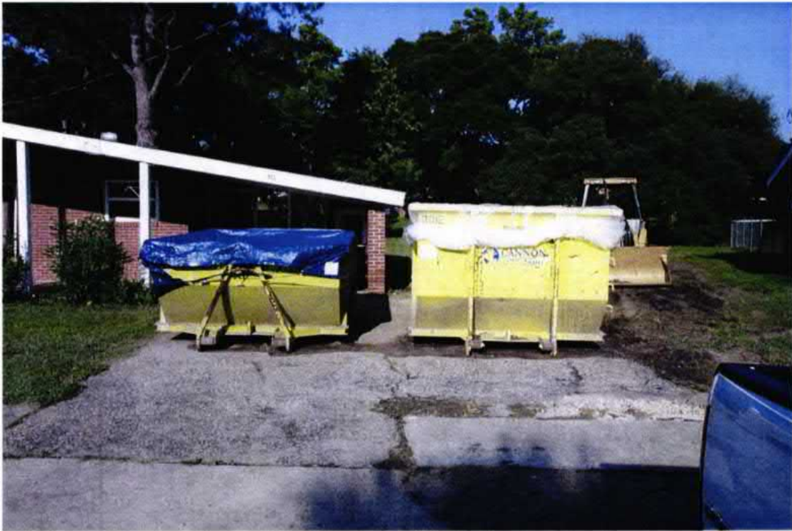
Excavated soil containment
