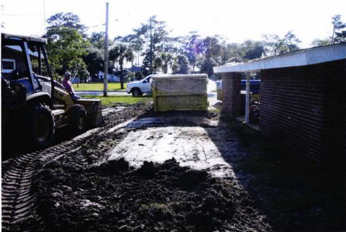
Fill dirt being spread over the excavation areas.
